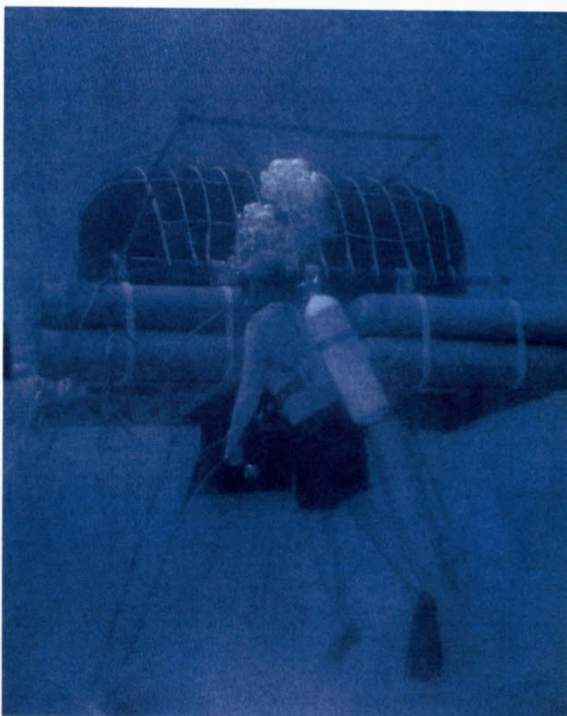
Figure 1: An underwater dwelling called the SPID (for "submerged, portable, inflatable dwelling") was designed by Edwin A. Link as a base of operations for long dives to the continental shelf, here undergoing a pressure test at 70 feet. In the summer of 1964 two divers occupied the SPID for two days at 432 feet below the surface.
